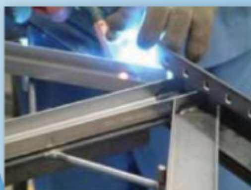
Welded assembly for main column
